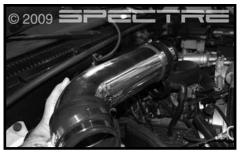
Step 15 Install the couplers onto both ends of the intake tube and secure with the supplied 4" hose clamps. Place the 3.5" hose clamps over the couplers and install the intake tube to the stock plenum and the filter assembly as shown.
